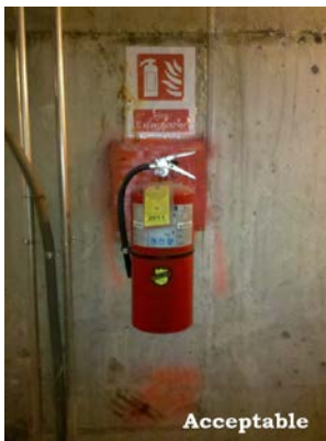
Fire extinguisher in a construction site.
